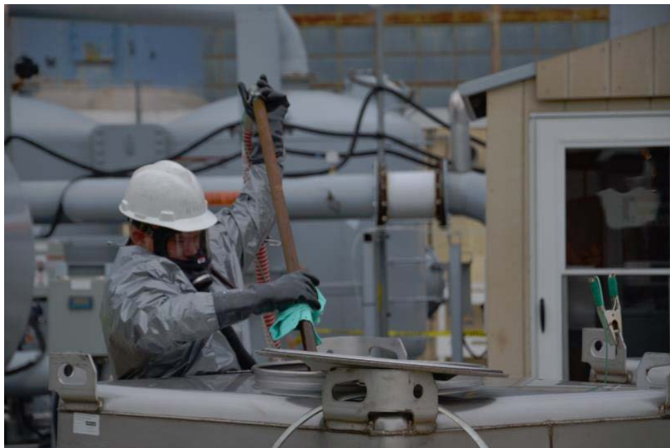
Figure 2.1 Remedial operations at the C-400 Cleaning Facility.
