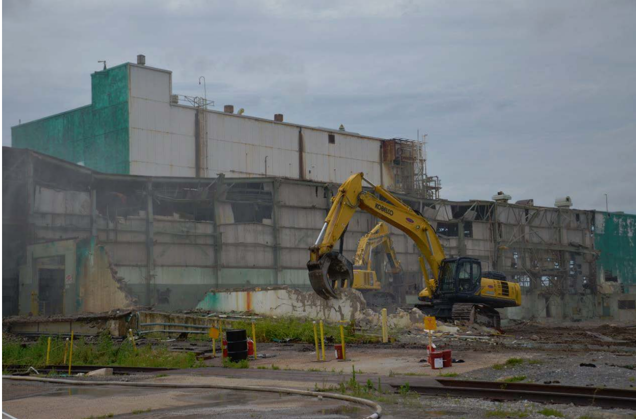
Figure 3.1 C-410/420 uranium feed plant building Demolition.
