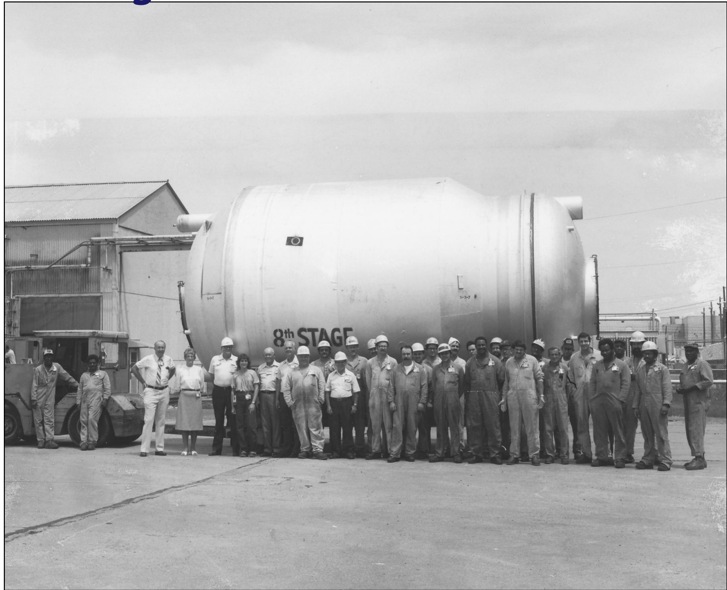
The 8 th Stage Compressor (of 1,760) from PGDP's diffusion process
