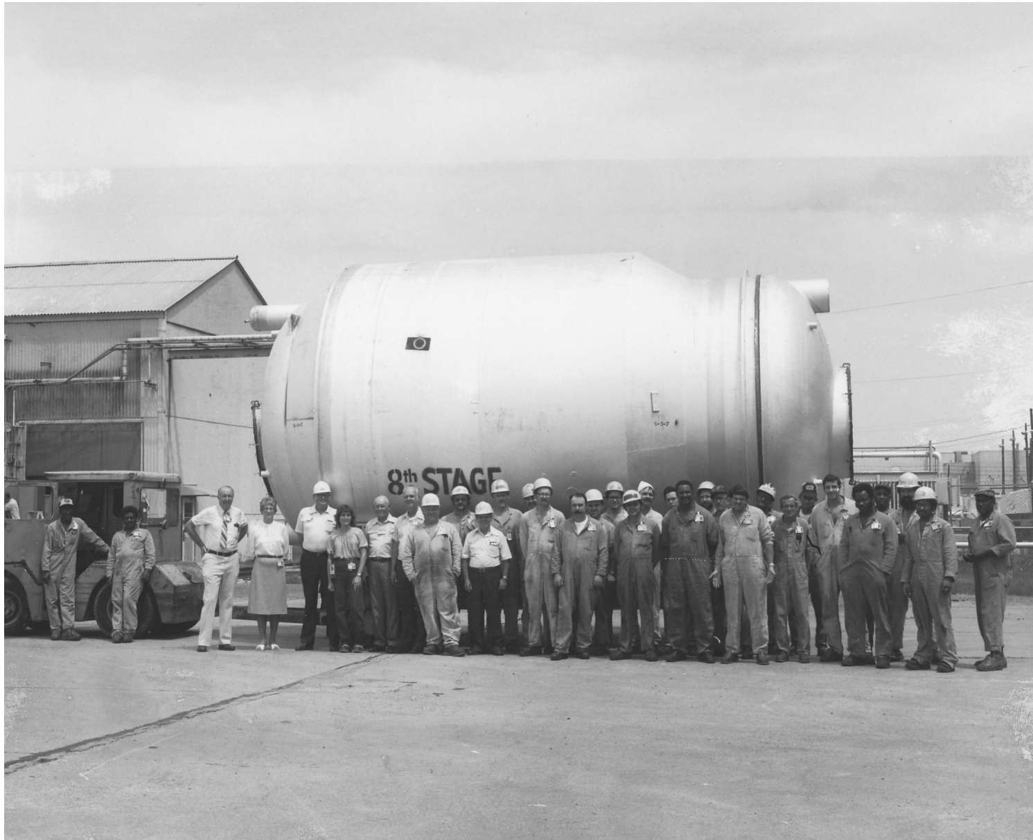
The 8 th Stage Converter (of 1,760) from PGDP's diffusion process
