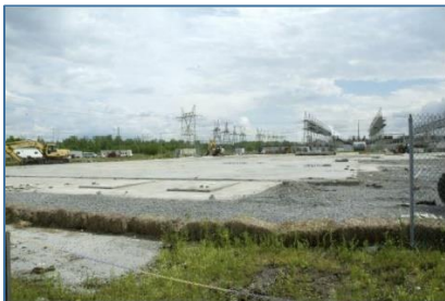
Figure 20. The C-340 Site following Demolition
