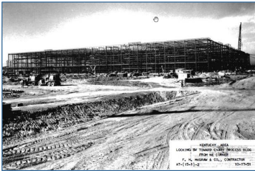
Figure 10. C-331 Early Construction
