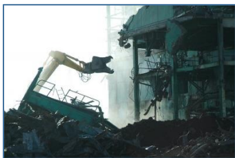
Figure 19. Demolition of C-340 Structures
