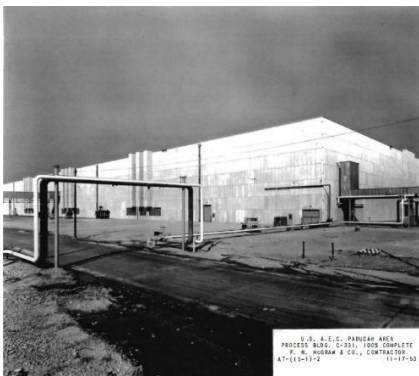
Figure 11. C-331 Process Building Completed
