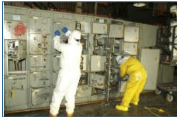
Figure 18. Workers deactivate C-340 Instrument Systems
