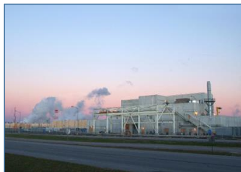
Figure 15. The PGDP DUF_6 Conversion Facility
