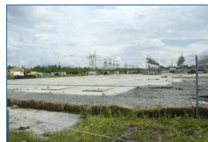
Figure 20. The C-340 Site following Demolition
