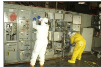
Figure 18. Workers deactivate C-340 Instrument Systems
