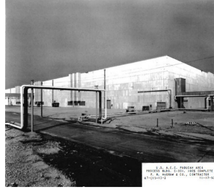
Figure 11. C-331 Process Building Completed
