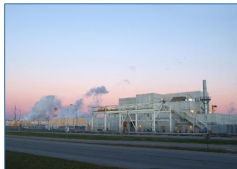
Figure 15. The PGDP DUF_6 Conversion Facility
