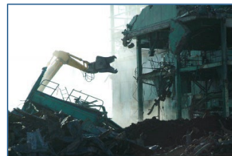
Figure 19. Demolition of C-340 Structures
